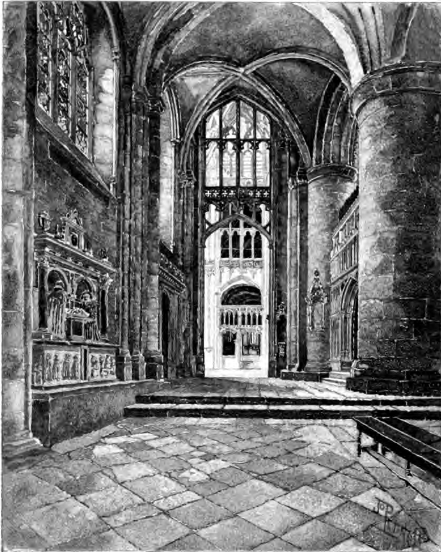
THE NORTH AISLE OF THE NAVE, LOOKING EAST INTO THE TRANSEPT.
